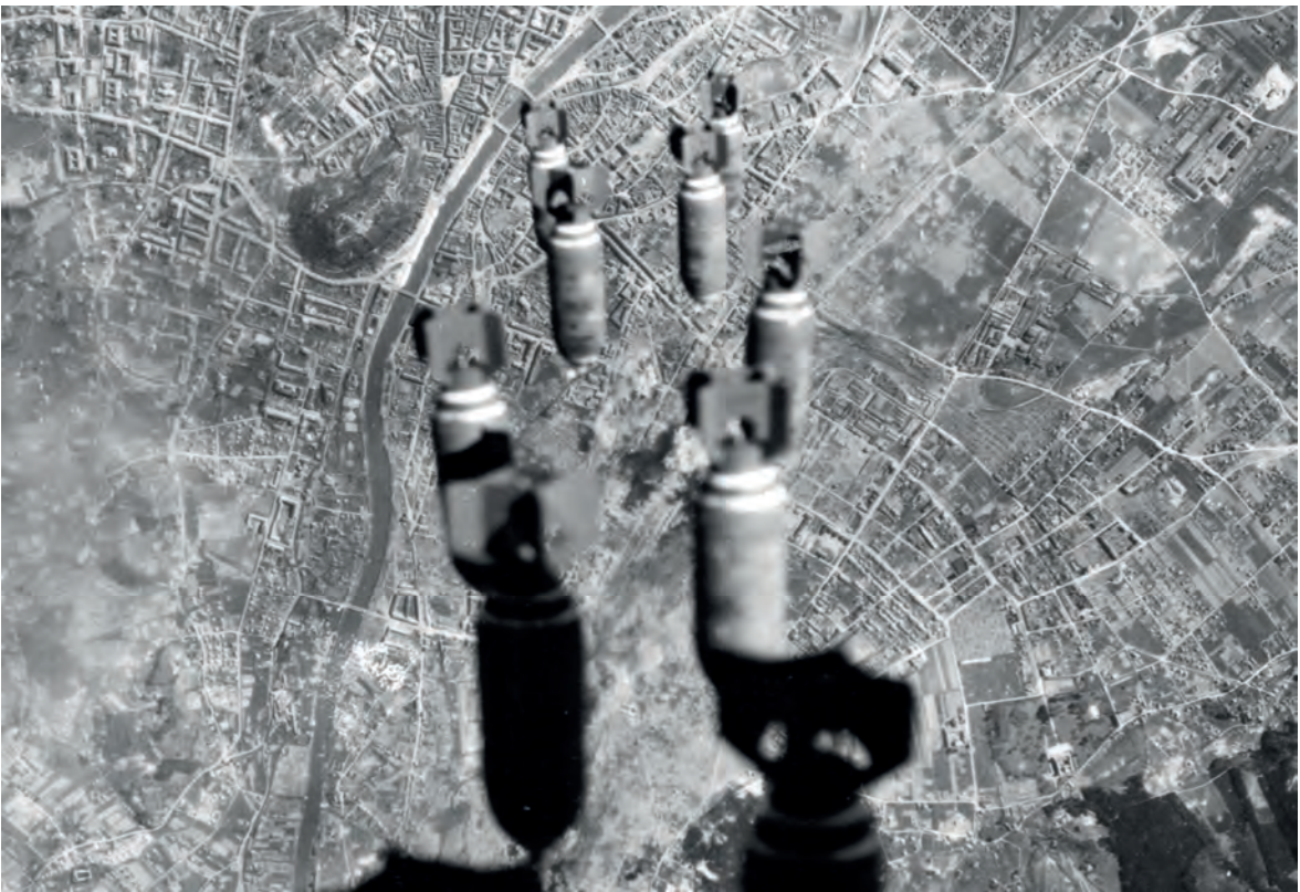
Bombs falling on the alternative targets of Klagenfurt, above, and Graz. (HF)
