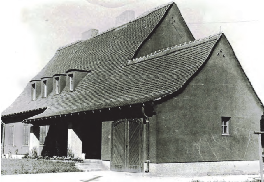
Villa built for the Plant Director Dr. Ing. Otto Judtmann, photo taken 1943 or 1944. Both director's homes and the single-family house had their own garage. [Doku STV]
