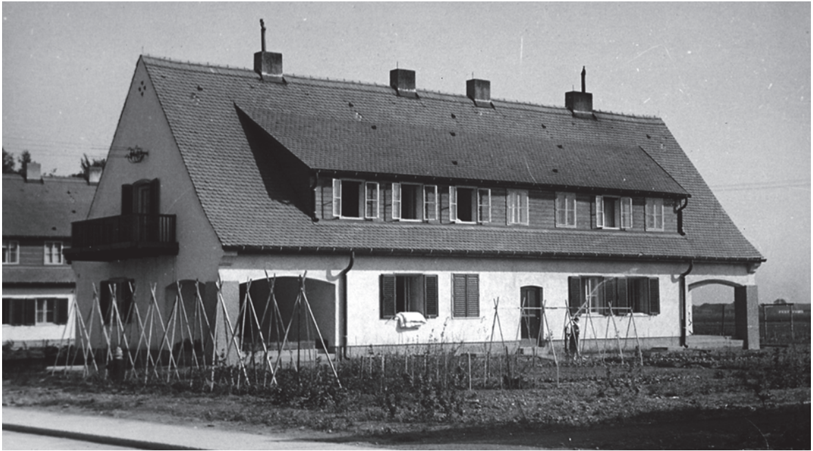
A typical type 4A apartment building (Herzograd 16). [Archive ECS]
