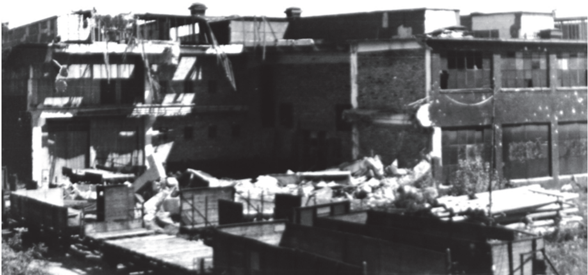
By the time the war ended, it was Workshop IV that was the least damaged. Only the north-west corner had been hit by a bomb. [Doku STV]
