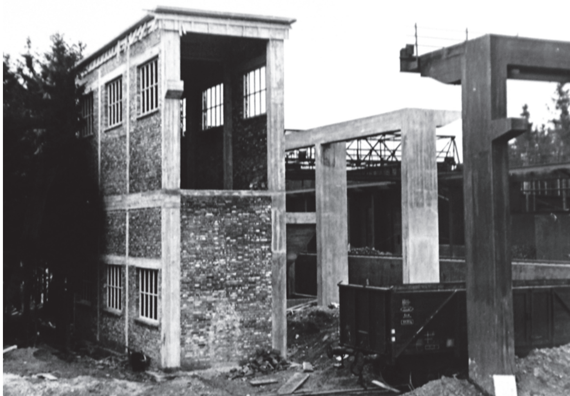
The completed and operational coal bunker for the boiler house in summer 1941. [Doku STV]
