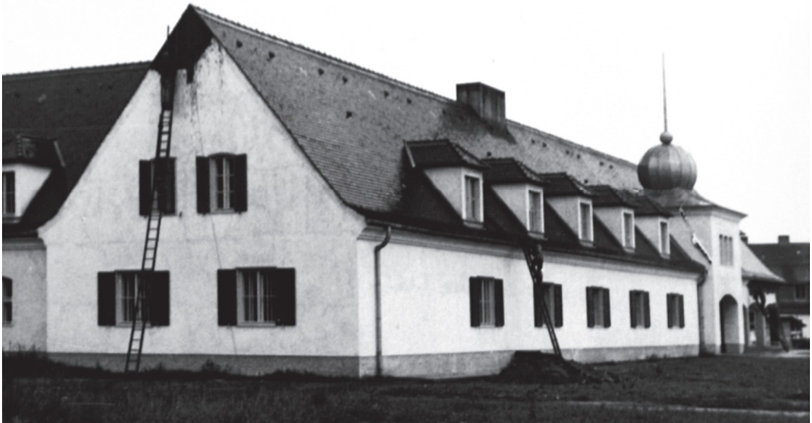
The staff home in the Herzograd residential development was painted a darker color in spring or summer 1943. [Doku STV]
