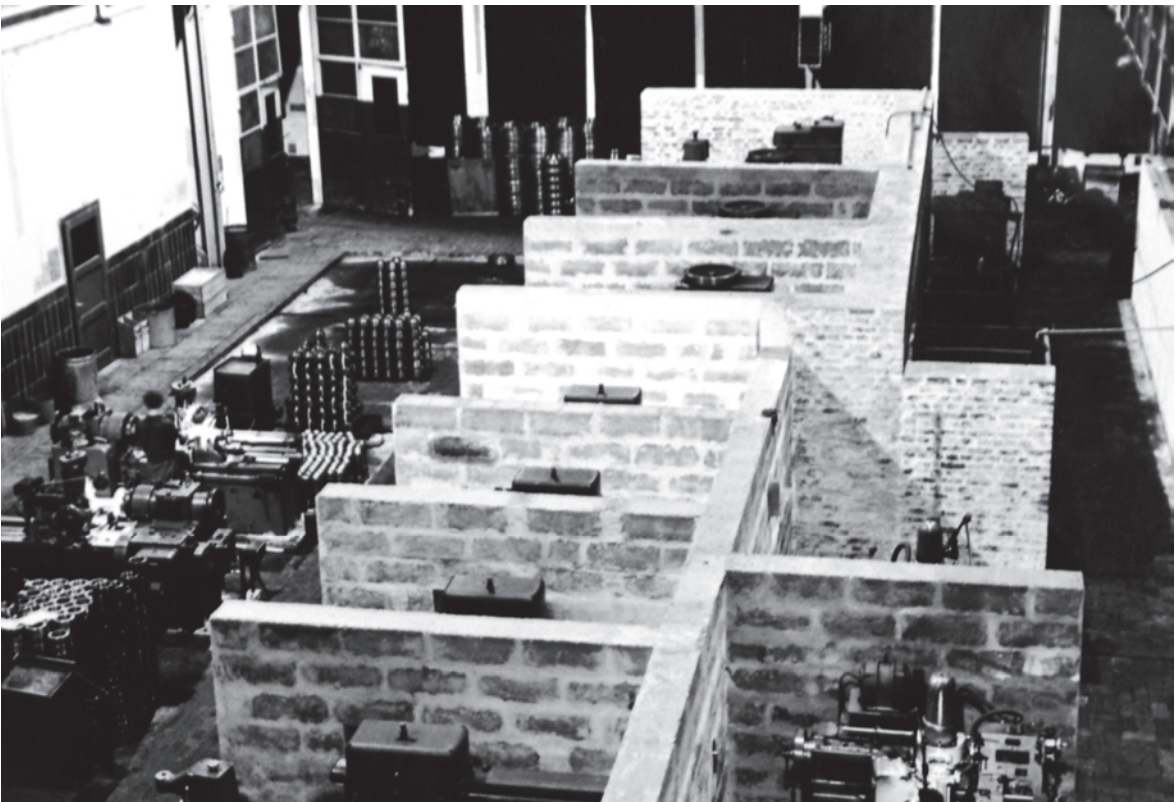
Blast walls made of engineering brick were built to protect the highly sensitive gear hobbing machines in Workshop I from shock waves and damage from bomb fragments. [Doku STV]
